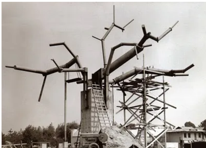
Figura 34 Estructura ramas principales Swiss Family Treehouse
